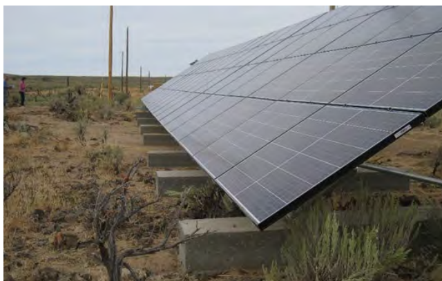
Solar installation as part of the Solar End-of-Feeder Pilot Project.
