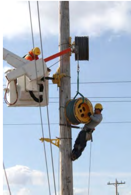
Idaho Power linemen install upgrades.
