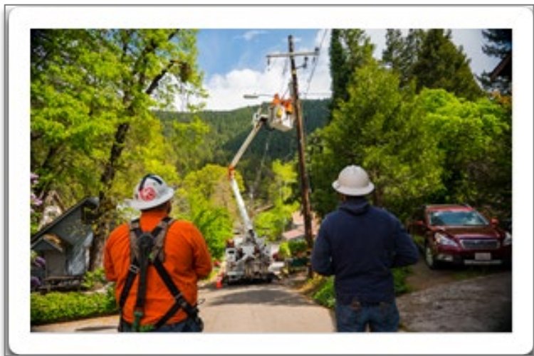
Figure 32: Line Workers Performing Work
