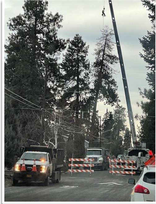
Figure 15: High-Risk Tree Removal
