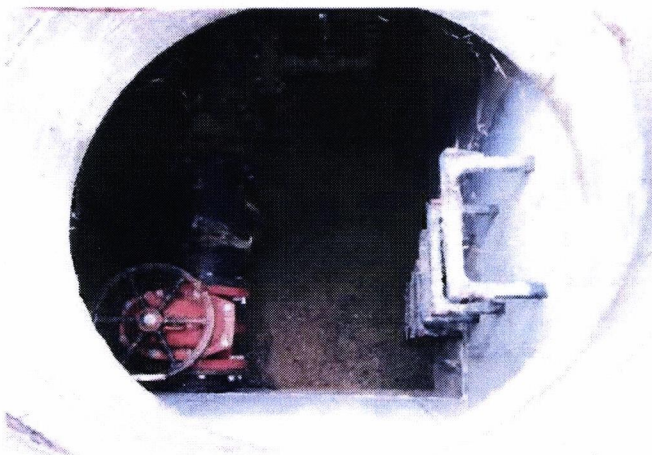
PRV vault access
