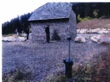
Well #1 and pump house
