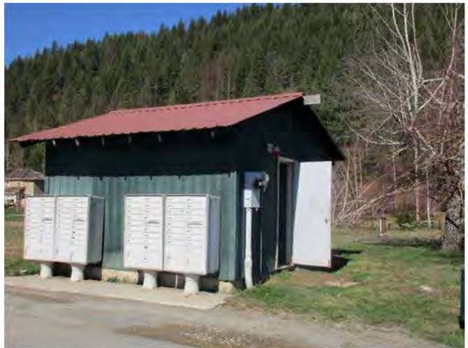
Photograph 6: Pump house for Wells 1 & 2
