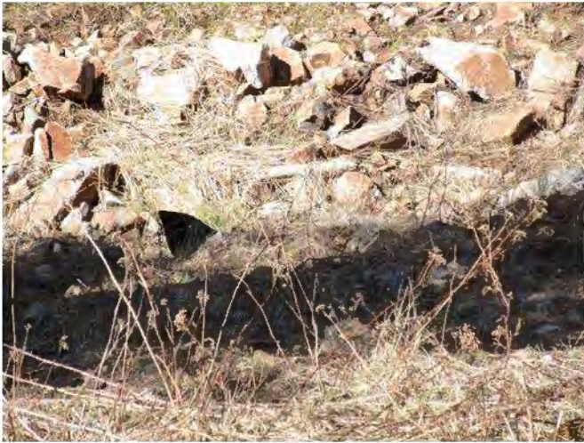
Photograph 69: SHST View downslope of drain flapper valve
