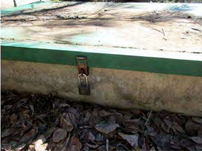
Photograph 25: MLST Locked hatch
