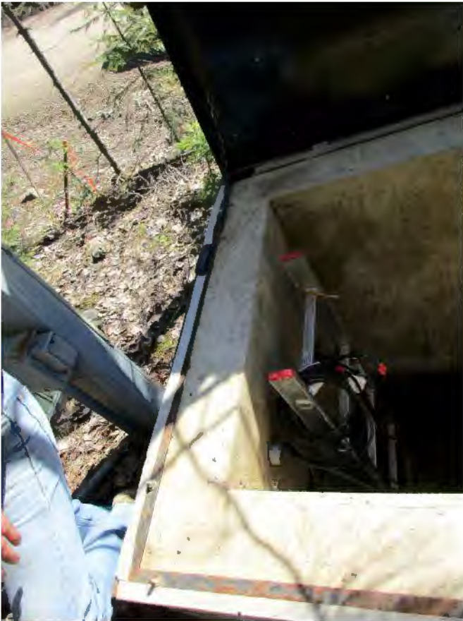
Photograph 29: MLST Hatch seal, concrete in good shape with no deterioration at
