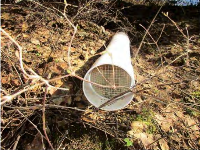
Photograph 39: Screened end flow to waste on UST
