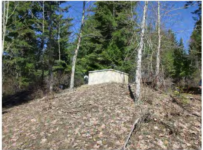
Photograph 30: View of upper underground storage tank (UST)
