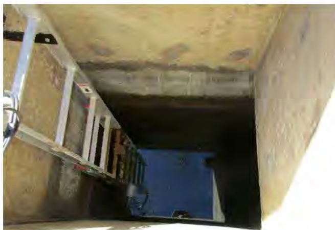
Photograph 34: View into UST, floats and ladder
