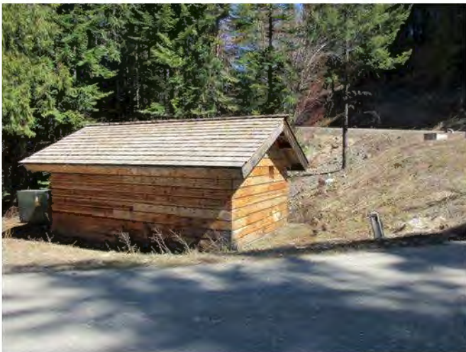
Photograph 55: Upper booster station (upper level) on southside of hwy
