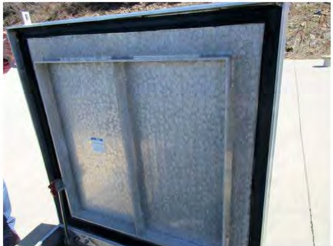
Photograph 66: Hatch seals in good condition
