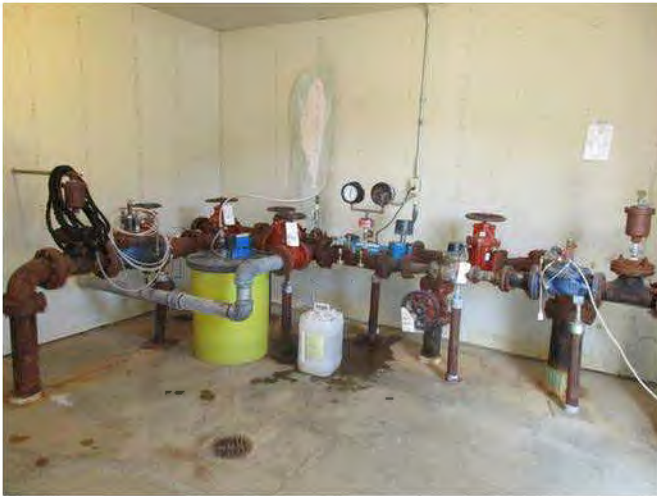
Photograph 7: Inside view of components of pump house
