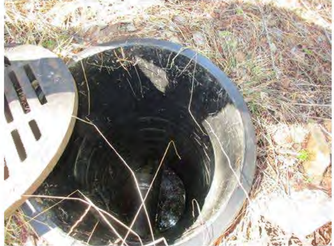
Photograph 52: Inside dry well drain (floor drain)
