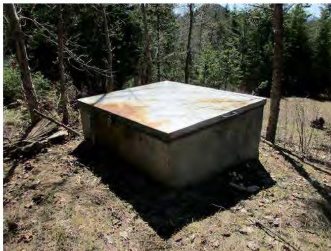
Photograph 32: Hatch riser on UST, locked with padlock
