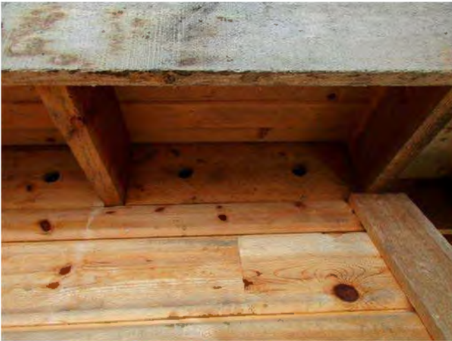
Photograph 43: Screened vent holes at roof line
