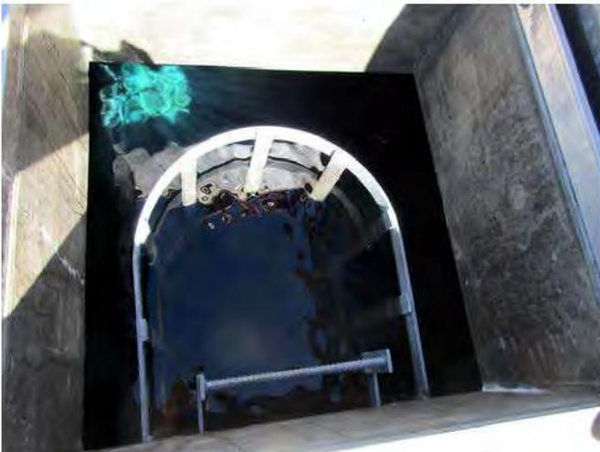
Photograph 65: View into one of 4 hatches
